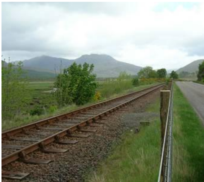
Road is alongside the Inverness to Kyle of Lochalsh railway line
