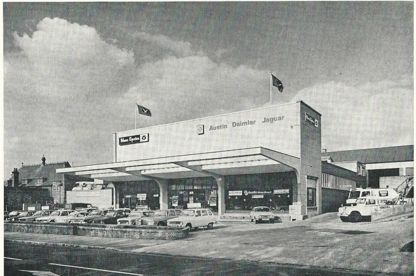
High Wycombe branch at London Road. Its barrel vault form of construction was one of the first in the country, allowing large uninterrupted floor areas.
