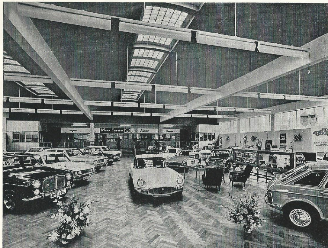
High Wycombe branch at London Road. Its barrel vault form of construction was one of the first in the country, allowing large uninterrupted floor areas.
