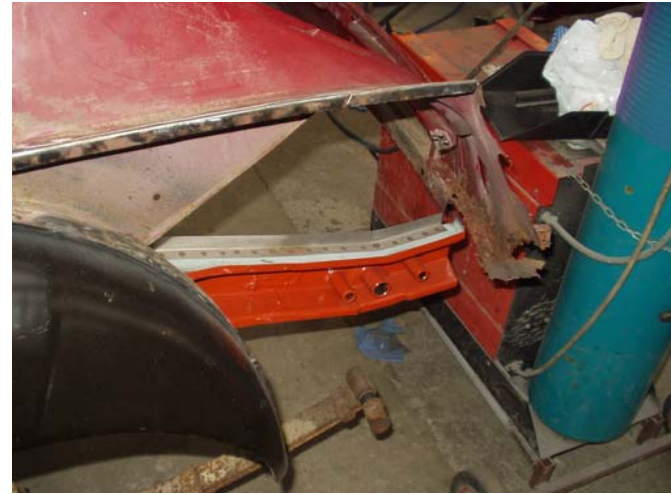
NSR spring hanger repair
