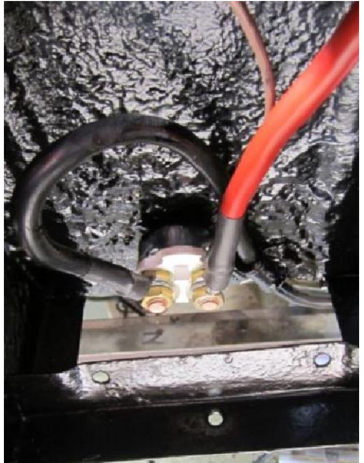
View looking down through the battery cover – the black cable runs from the new switch under the car and forward to the starter motor. The thinner brown wire runs into the car and forward along the tunnel to provide a permanent (unswitched) supply to the radio.
