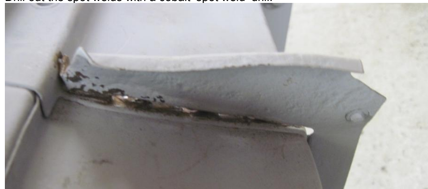
Use a chisel to start breaking the rusty part away from the top of the inner wing. Any comments, suggestions to mikemacartney@btconnect.com 18 th June 2016
