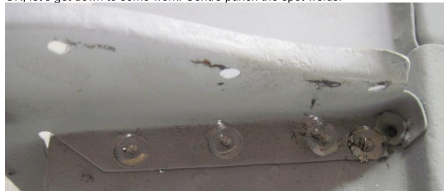
Drill out the spot welds with a cobalt 'spot weld' drill.
