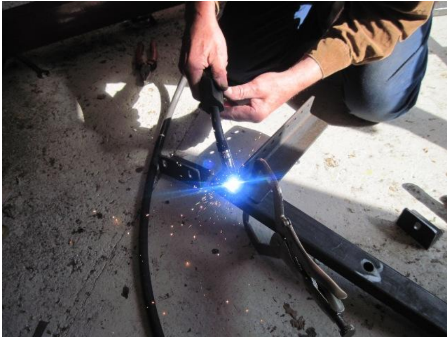
Clamped at right angles and tack welded.
