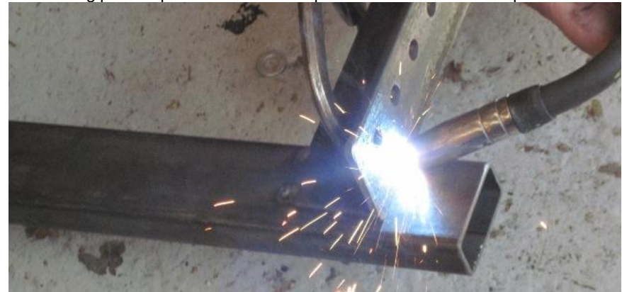
Tack welding the bits of spit together.
