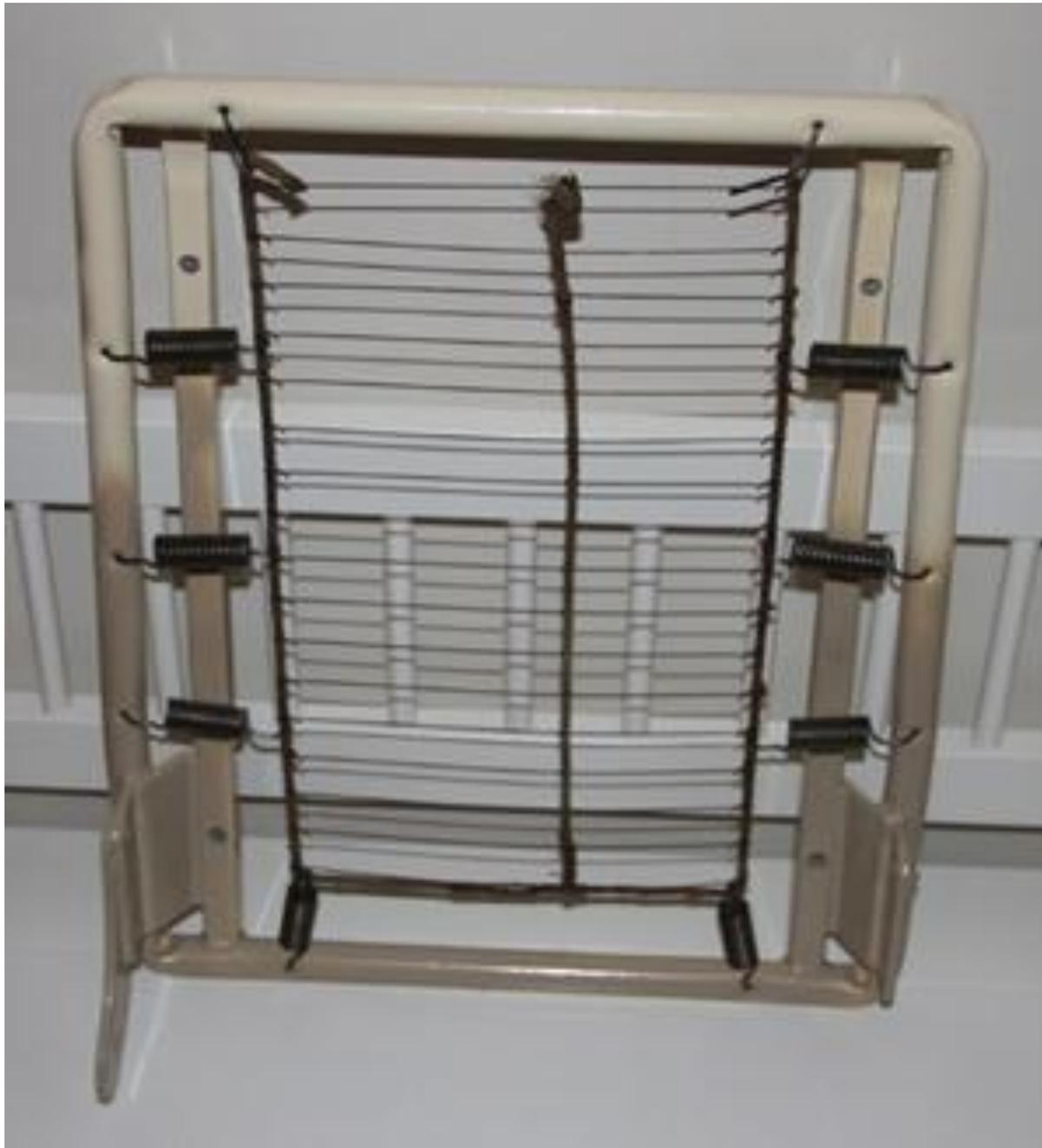
back is attached to the back frame. The back frame needs to be sanded (I used a DREMEL) then painted with primer and spray painted with Motip 46400.
