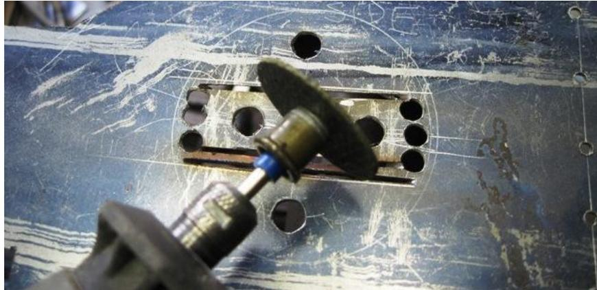
Cutting the centre out for the battery cut off switch
